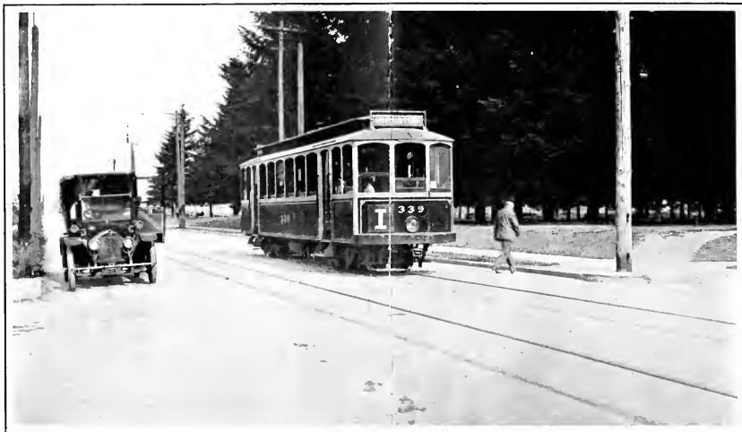
Hassam Pavement on Multnomah Street, Portland, Oregon. Holladay Park at the Right has "Hassam" on Four Sides
